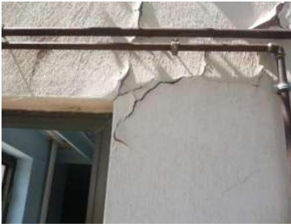
Figure 8. The cracks in column-beam connections
