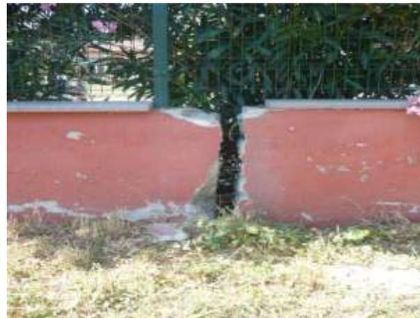
Figure 6. Separations in walls due to soil movements
