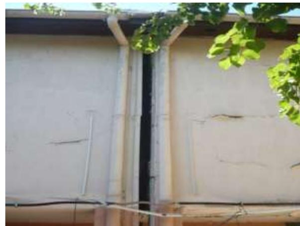
Figure 7. The separation in dilatation joints
