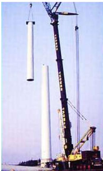
Fig. 4 Nordex N43 tower during construction.
