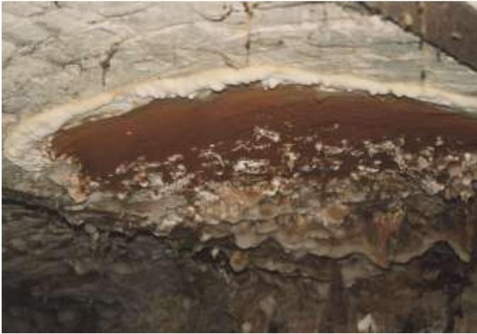
Fig. 5. The fruiting body of the house fungus proper (*Serpulla lacrymans*), grown into a vaulted ceiling of a basement room
