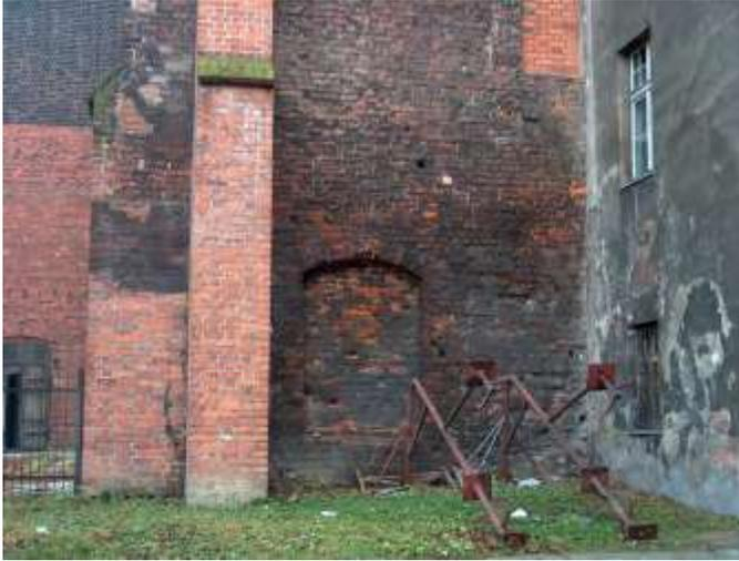
Fig. 3. Moisture level of the northern wall reaches approx. 5 m high above ground level - Museum in Raciborz.
