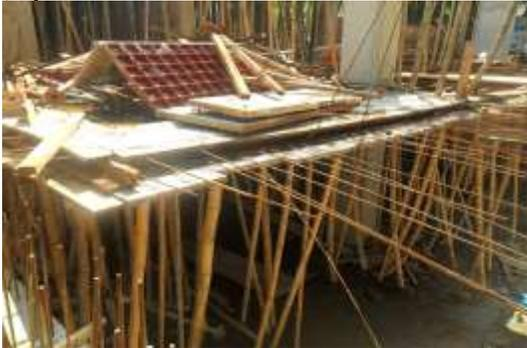
Figure 2. Bamboo props used as scaffolding and no safety net is present (may cause accidents to the pedestrians)
