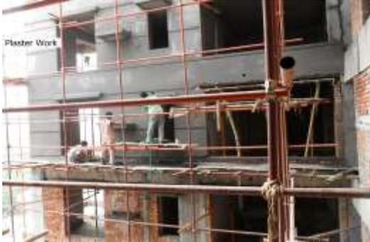
Figure 1. Workers working without any safety precaution (may cause fall accidents to the workers)
