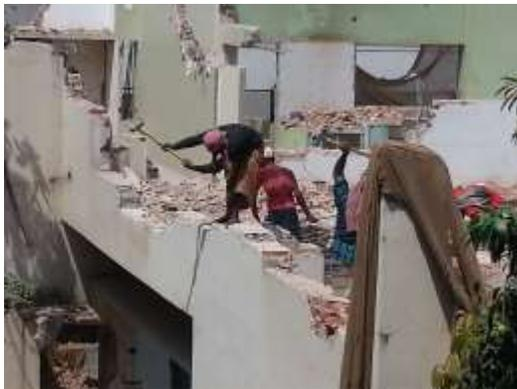
Figure 4. Unsafe condition during demolition work
