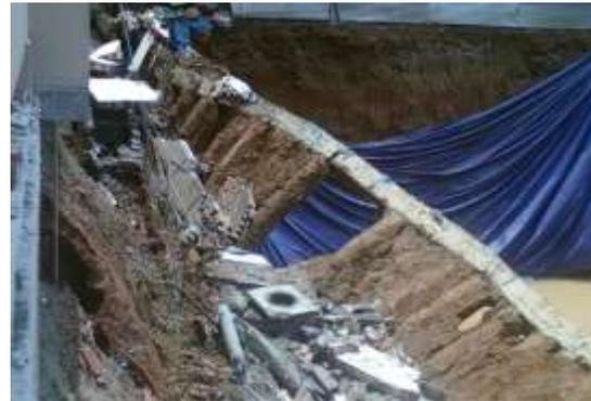
Figure 3. Trench collapse on a construction site
