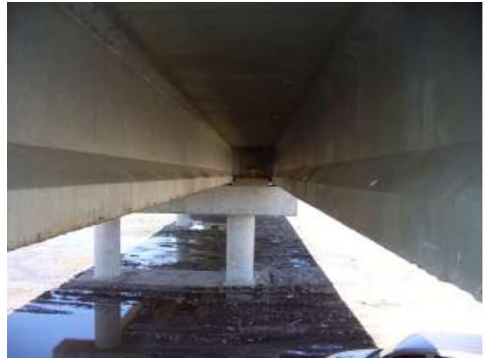
Figure 12. View of the damper. Bridge in Sorocayense, San Juan-Argentina
